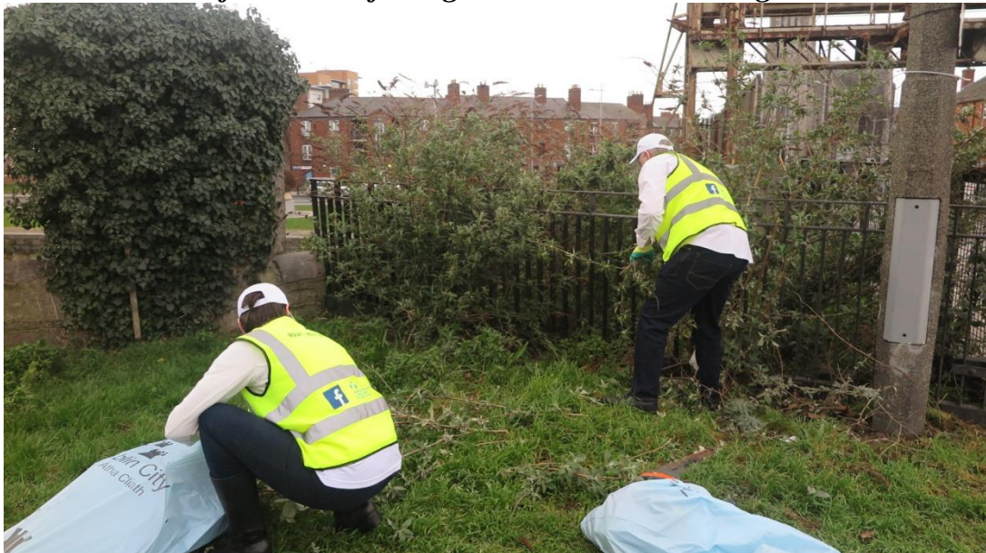
Before East facing south side Samuel Beckett Bridge
