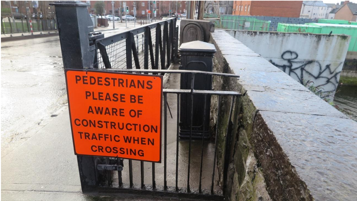
After on North side of Samuel Beckett Bridge
