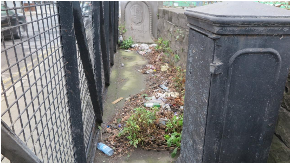
Before on north side of Samuel Becket Bridge
